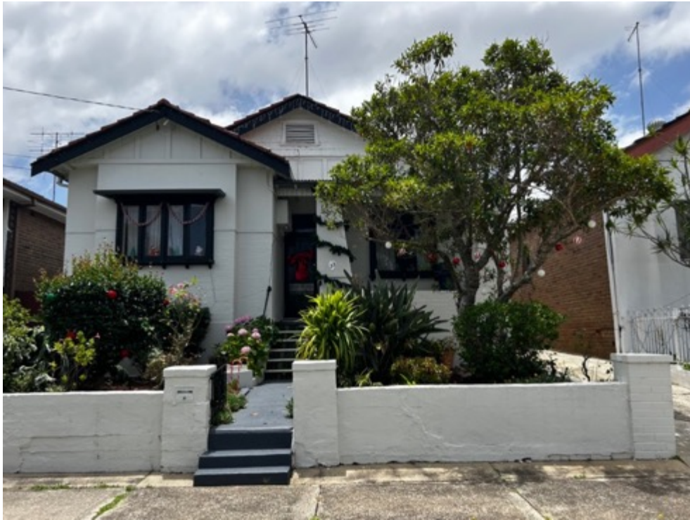
Photograph 1: Street (South) Elevation: full frontage, taken from Third Street
