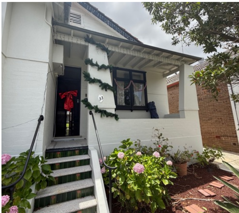
Photograph 2: Front Verandah and Entry Detail
